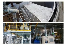
Above. Dissolved Air Flotation installed at the paint shop 52 of the Ulsan Plant Below. EVs installed at the industrial water treatment facility of the Asan Plant
